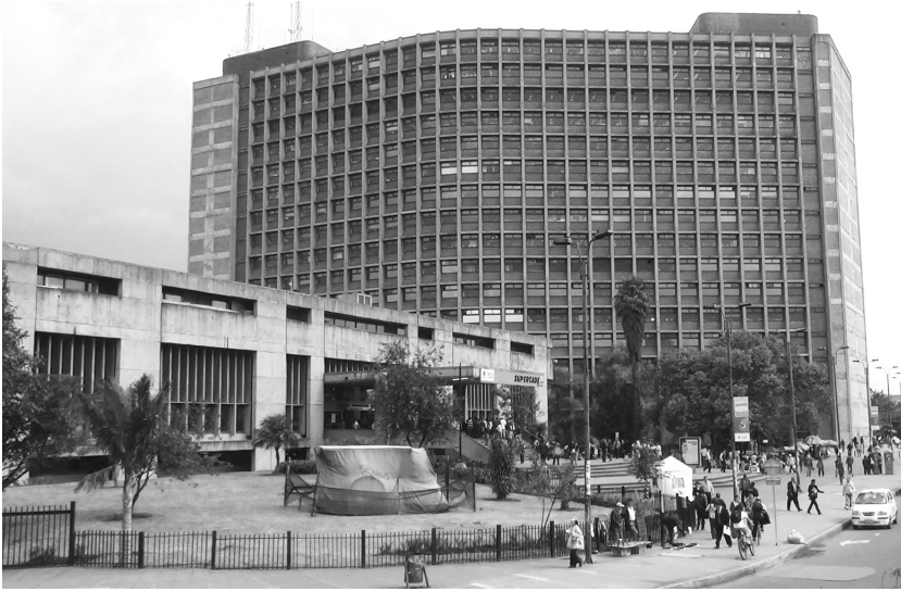
Figure 5.1. The Secretaría de Planeación and the citizen service center building where the Grupo POT's office was located. Photograph by Federico Pérez.
